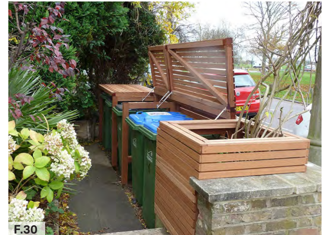
Figure 30: Waste storage along the boundary treatment.
